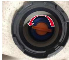
Turn Filters Counter-clockwise to Remove
