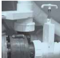
Slice Valve and Pump Union
