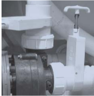
Slice Valve and Pump Union
