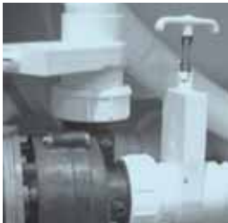
Slice Valve and Pump Union
