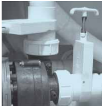
Slice Valve and Pump Union
