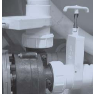
Slice Valve and Pump Union
