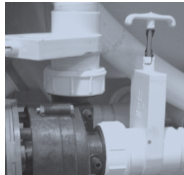
Slice Valve and Pump Union
