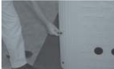
Removing of Panels
