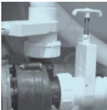
Slice Valve and Pump Union
